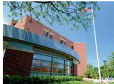
NorthShore Highland Park Hospital
