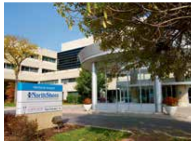
NorthShore Glenbrook Hospital
