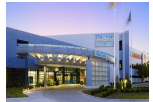
Skokie Hospital 9600 Gross Point Road Skokie, IL 60076
