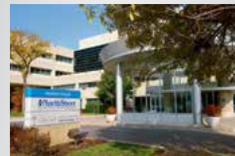
NorthShore Glenbrook Hospital
