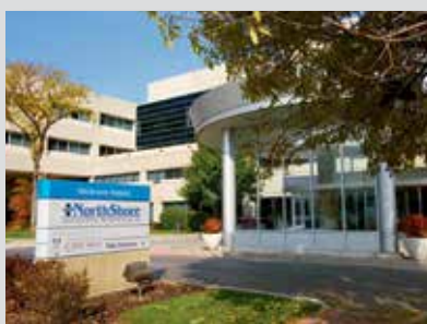
NorthShore Glenbrook Hospital
